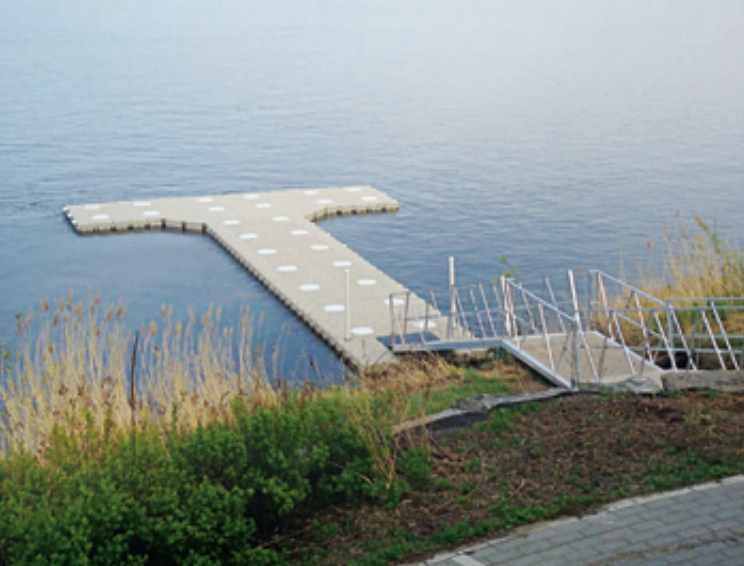
PUBLIC ACCESS FLOATING DOCKS
