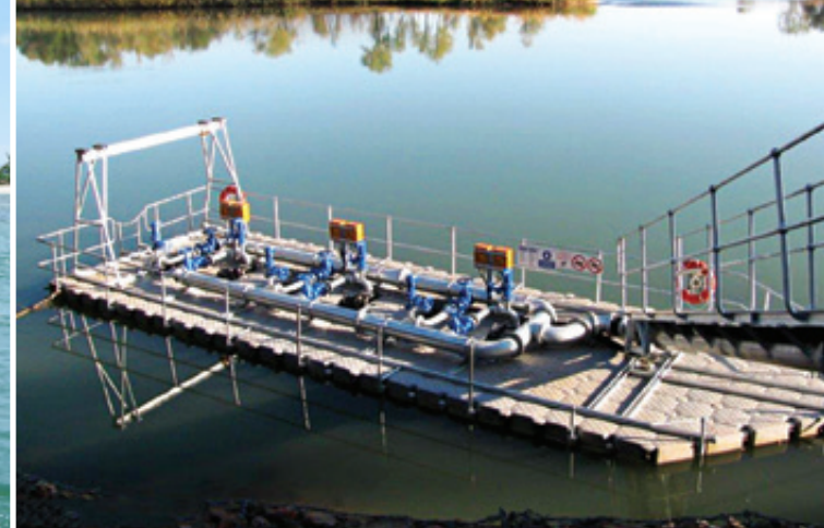
WATER PUMP INTAKE PLATFORMS
